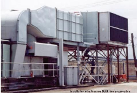
Installation of a Munters TURBIdek evaporative cooling system increased power output by 2.4 MW.
